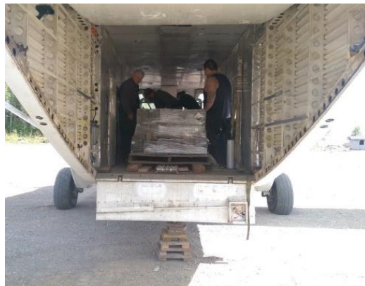
Lead battery removal
