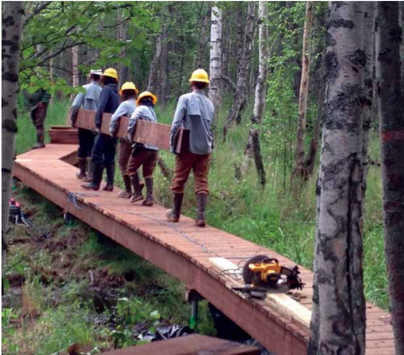
Great Land Trust partnered with the Student Conservation Association to build a light penetrating wetland boardwalk that provides an easy way for people to experience the Palmer Hay Flats Game Refuge. Kim Sollien/Great Land Trust
