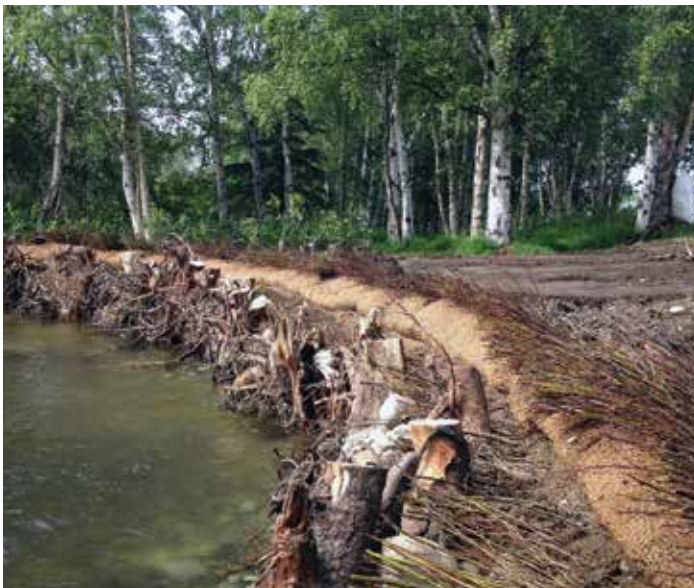
Restoring streambanks on Wasilla Creek. These vegetated shoreline areas provide cover for juvenile fish; cooler temperatures; have slower moving currents where weaker swimming fish can rest; and have over-hanging plants that fall into the water, creating food sources for aquatic insects that juvenile salmon eat. Photos: Frankie Barker/Mat-Su Borough and Jessica Speed/The Nature Conservancy
