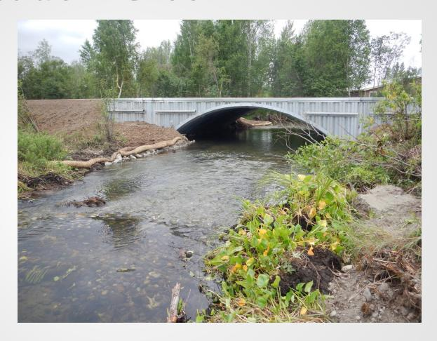
After: 32'-0" x 10'-0" Bottomless steel low-profile box culvert with headwalls and wingwalls
