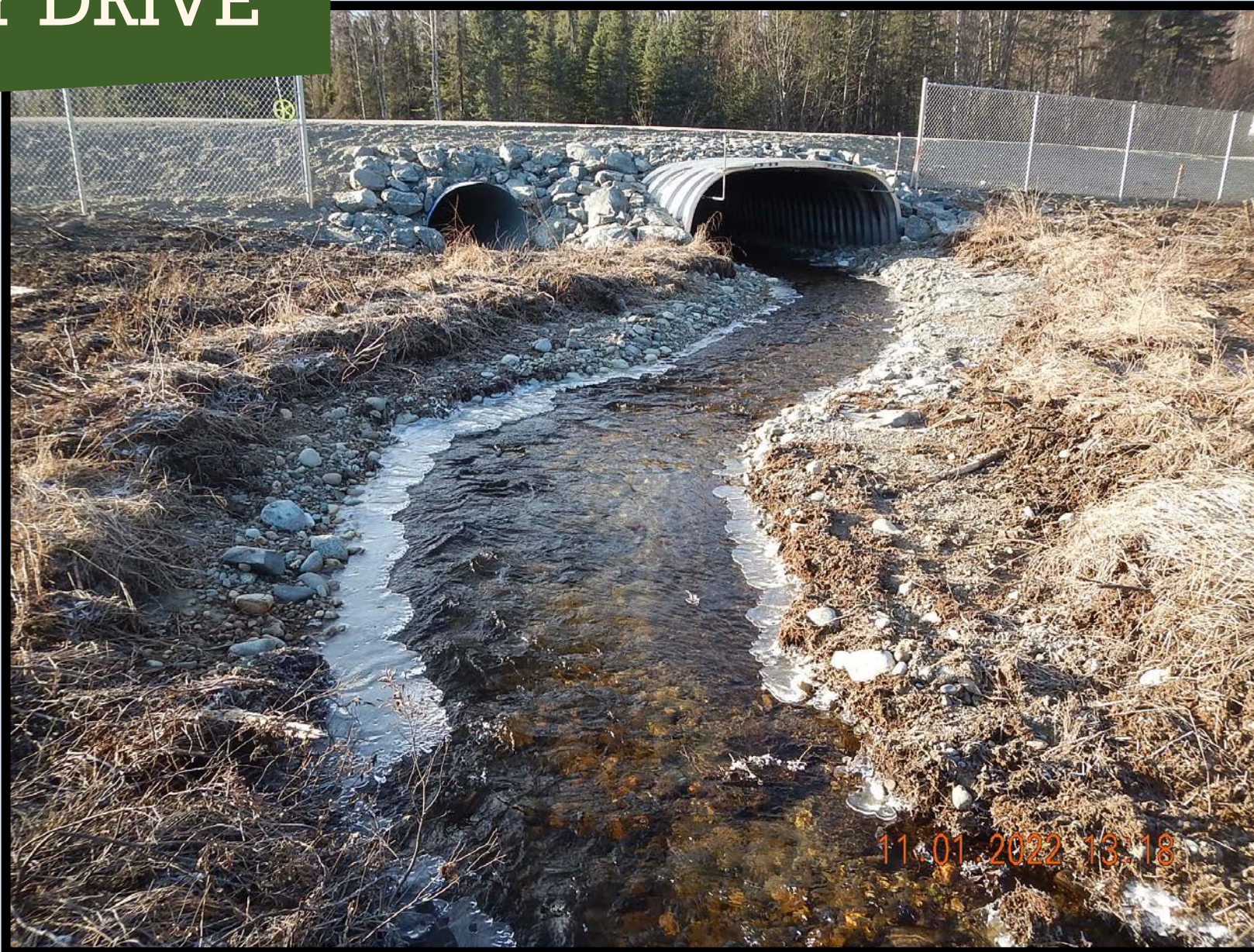
Photo: Upstream view and new inlet.
