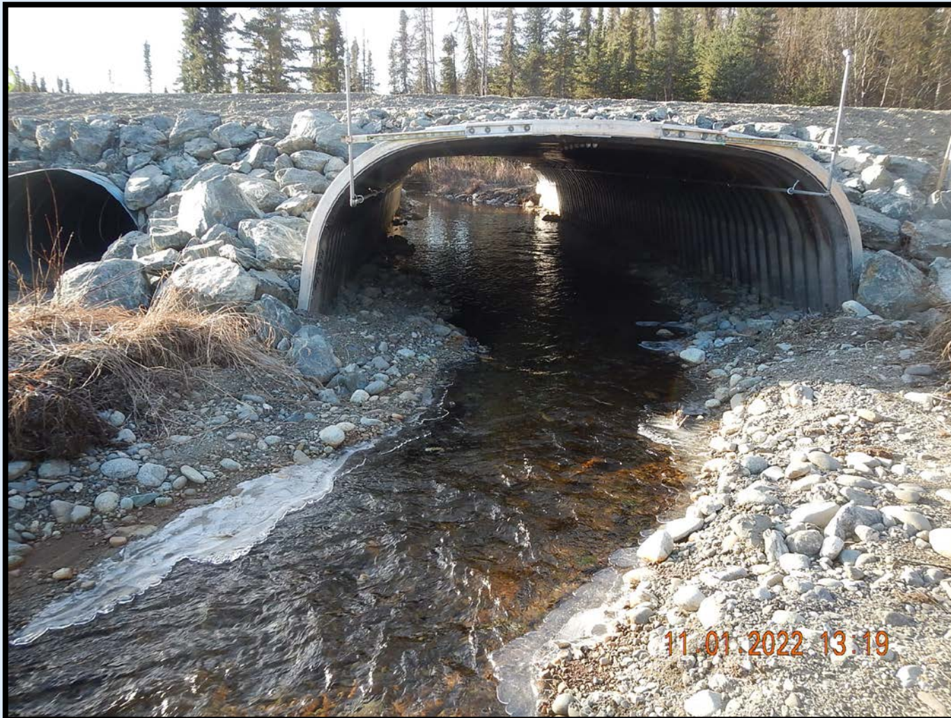
Photo: Newly constructed inlet.
