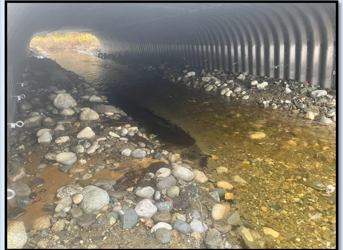
Photo: Constructed streambed inside the culvert.
