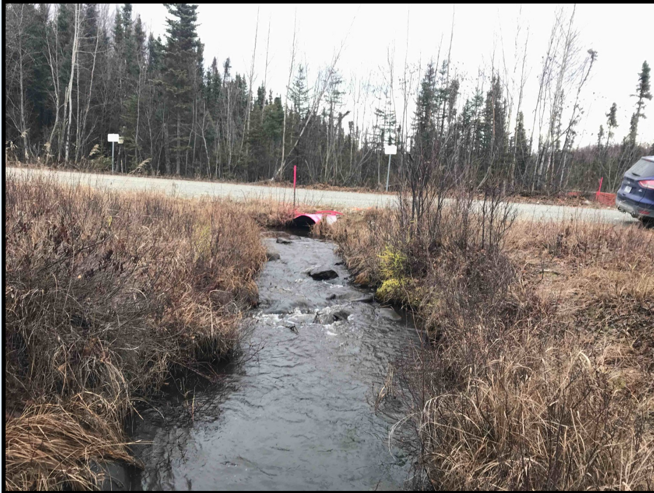
Photo: Existing culvert outlet.
