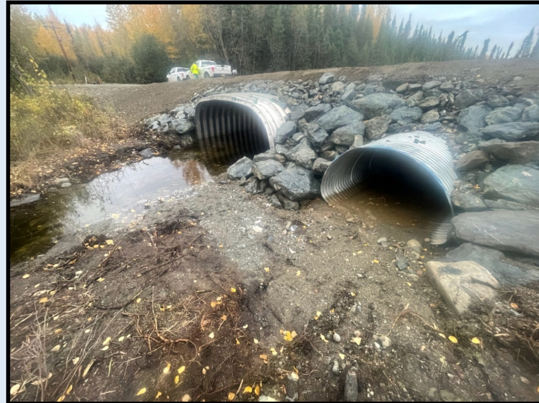
Photo: New culvert and floodplain culvert outlets.
