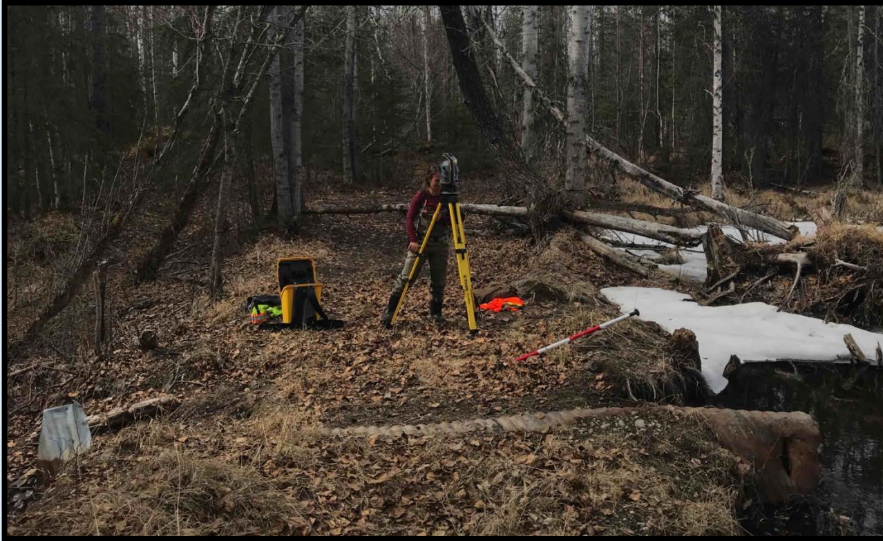
Photo: Surveying existing conditions.
