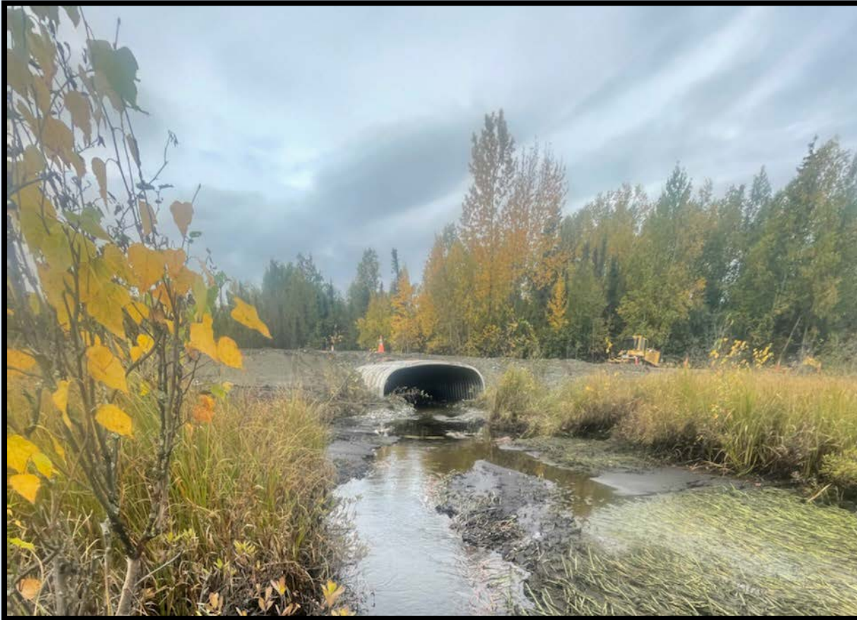
Photo: New culvert inlet.
