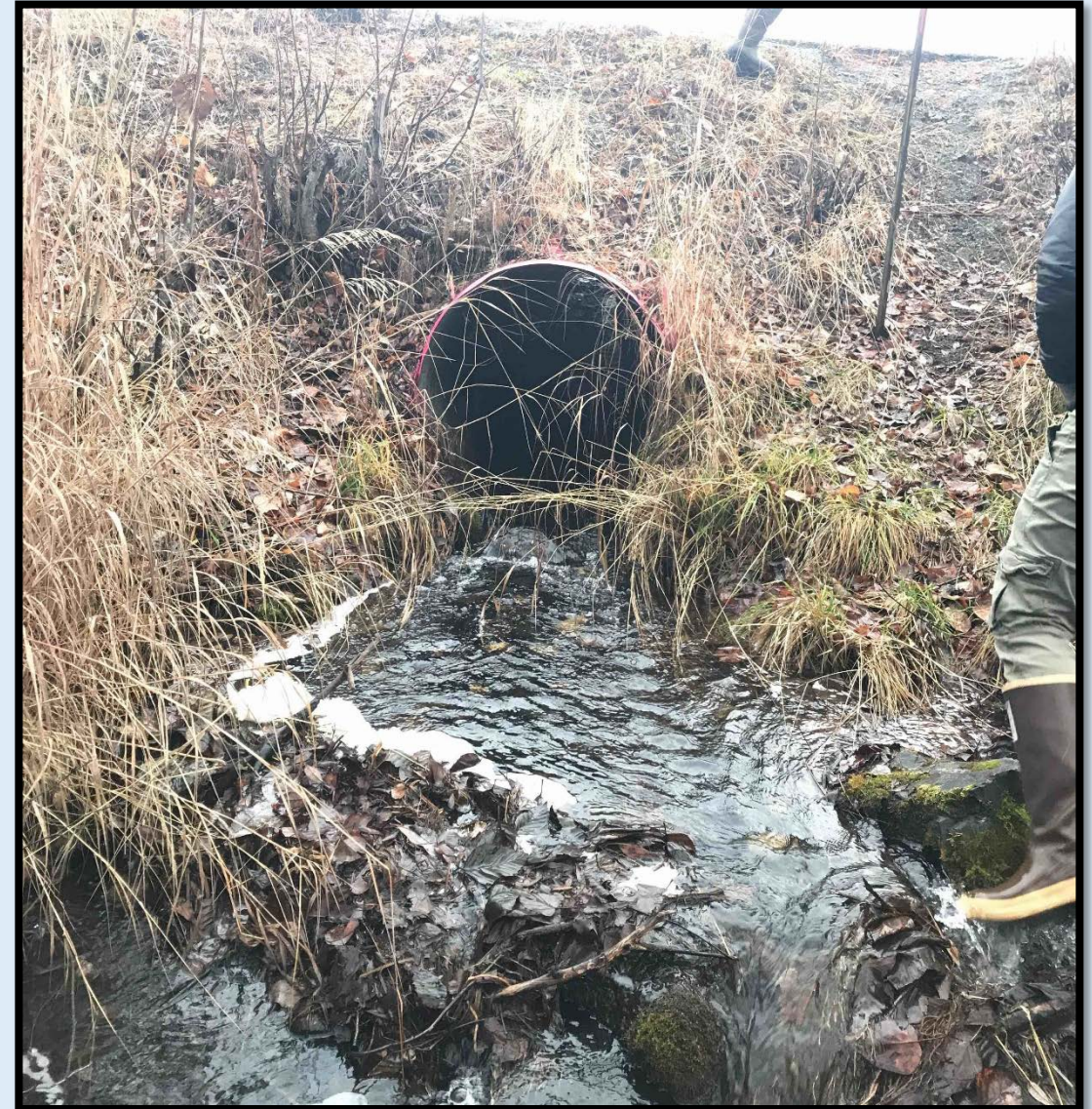
Photo: Existing culvert outlet.
