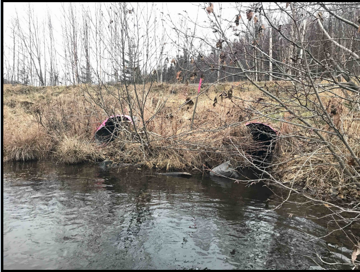
Photo: Existing culvert inlet.
