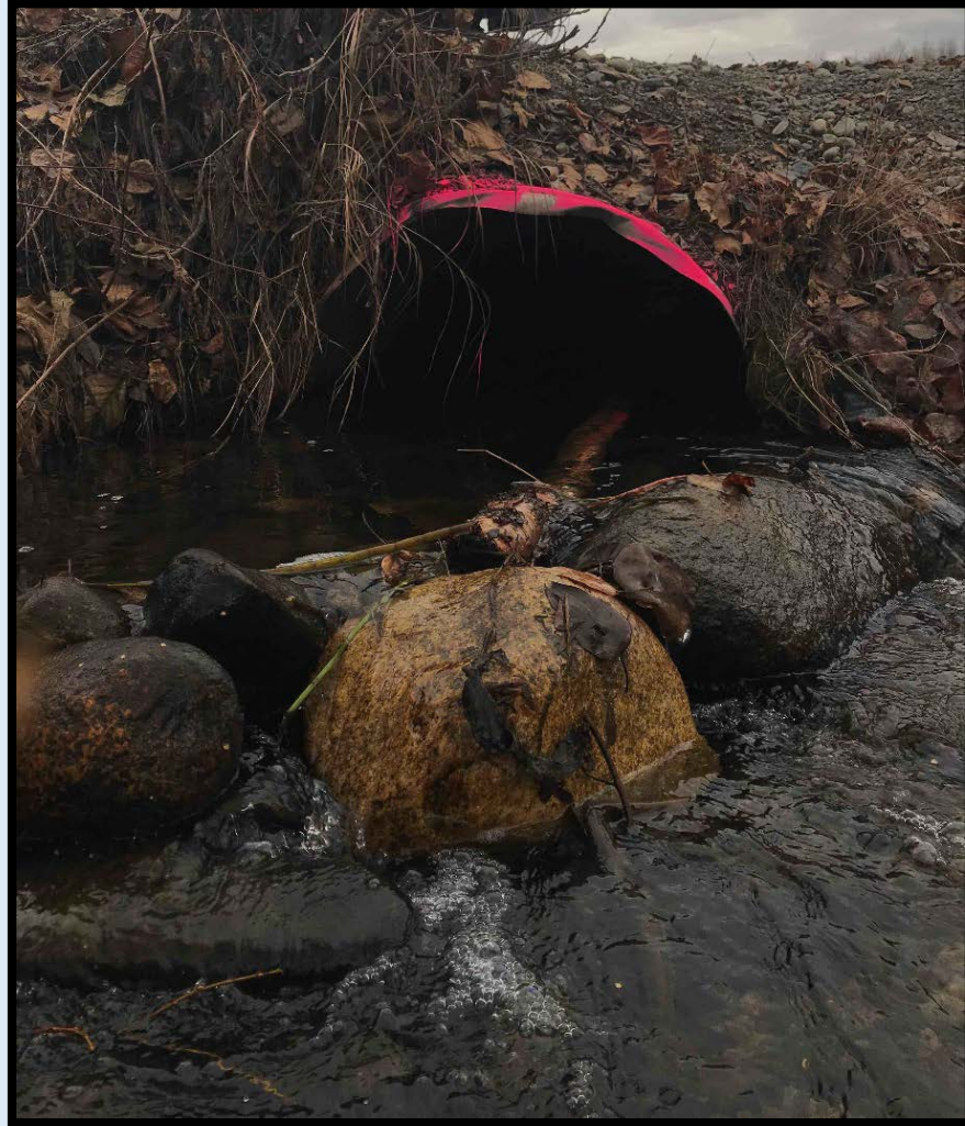
Photo: Existing culvert outlet.
