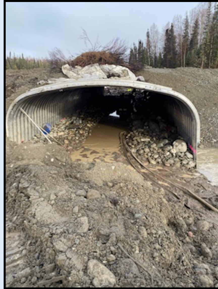
Photo: Streambed installation.
