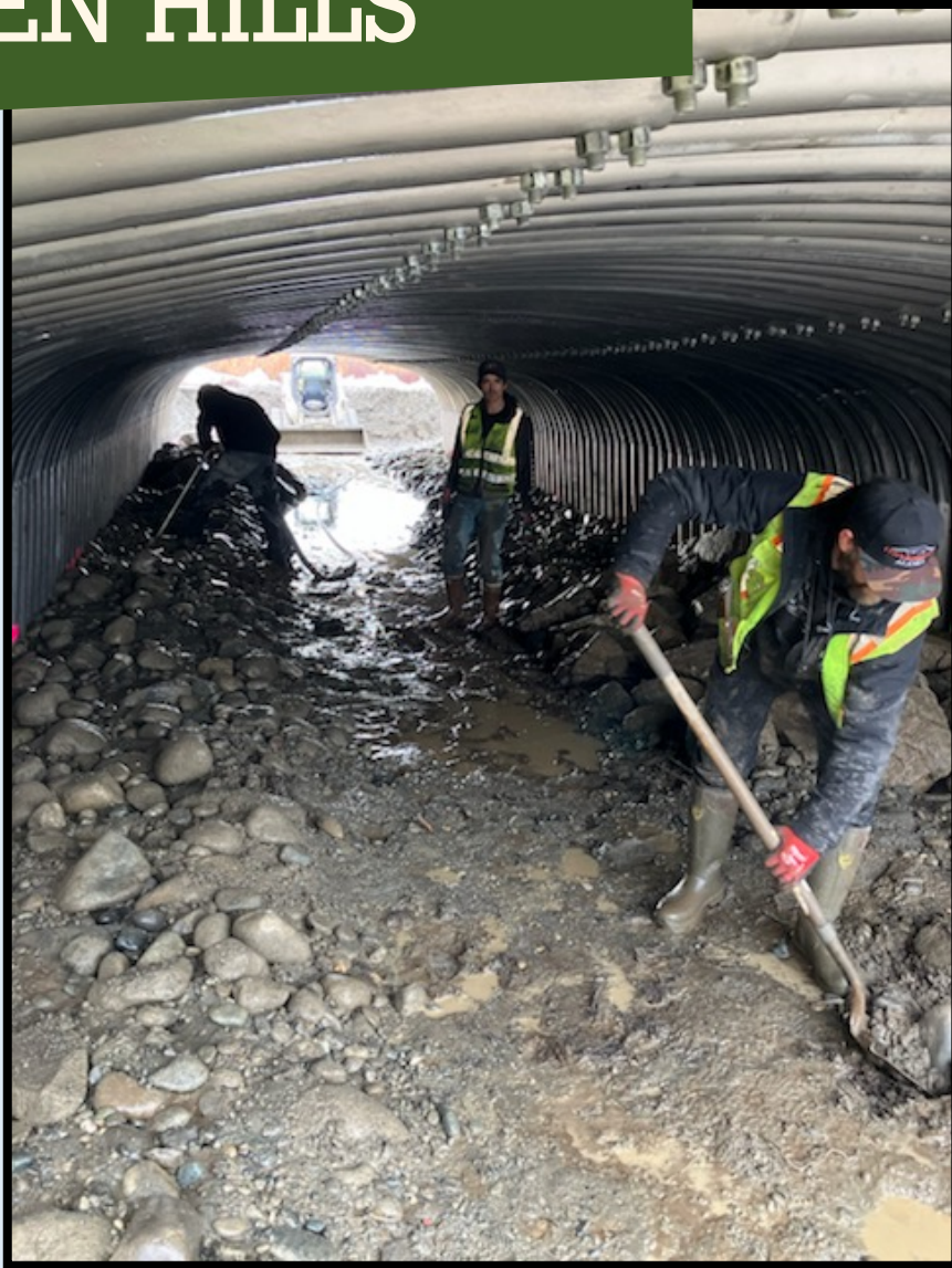
Photo: Construction of streambed.
