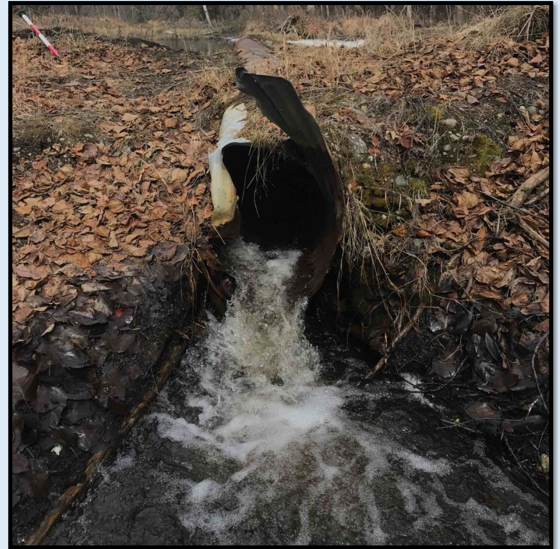
Photo: Culvert outlet.
