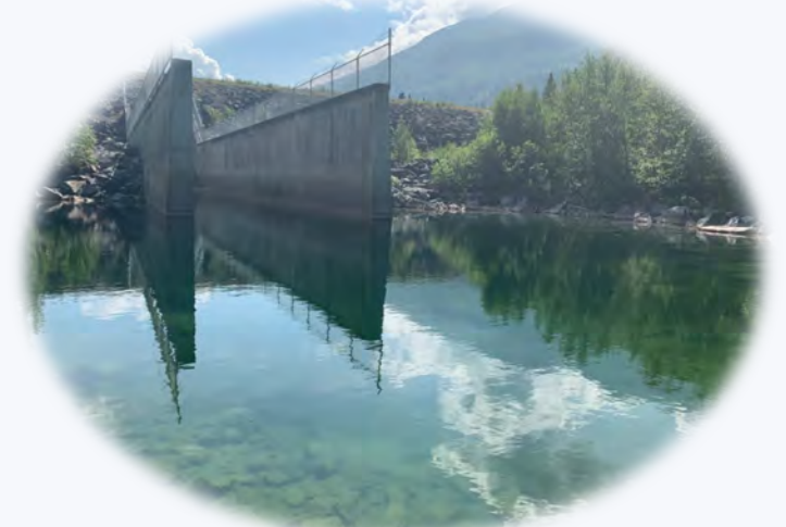
Eklutna Lake Dam, looking upriver
