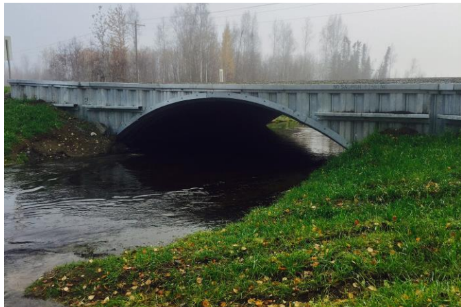
Meadow Creek at Beaver Lake Road – completed
