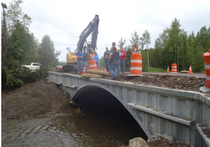
Construction on Meadow Creek, summer 2015
